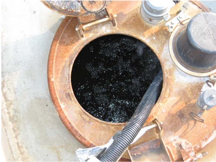
Oxygenated Feed Water Return to Tanker
